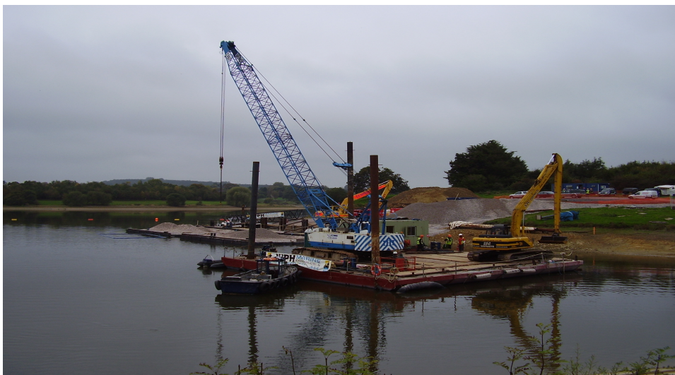
Figure 7 - Plant and barges for underwater work
