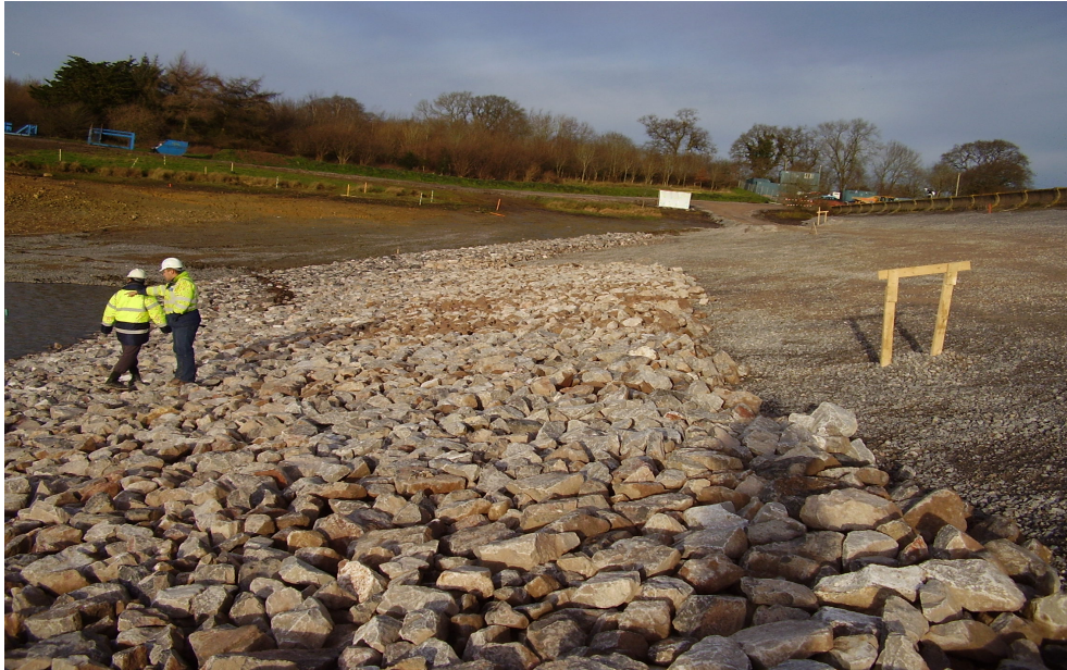
Figure 6 - Recently placed rip-rap Underwater Works
