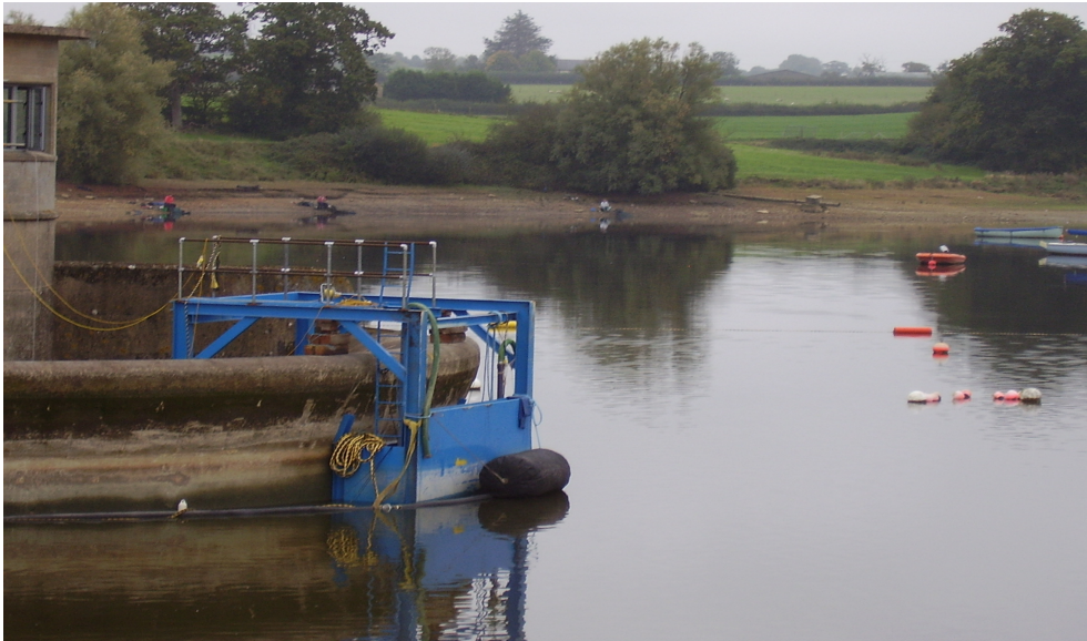
Figure 1- Limpet type cofferdam
