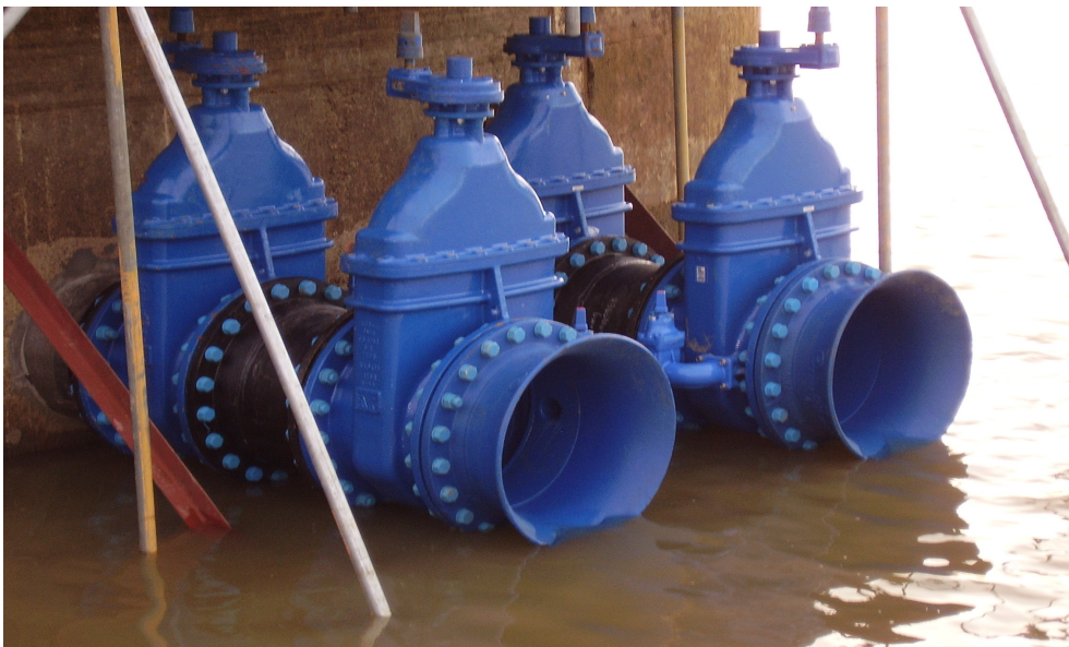
Figure 2 - New bottom outlet valves
